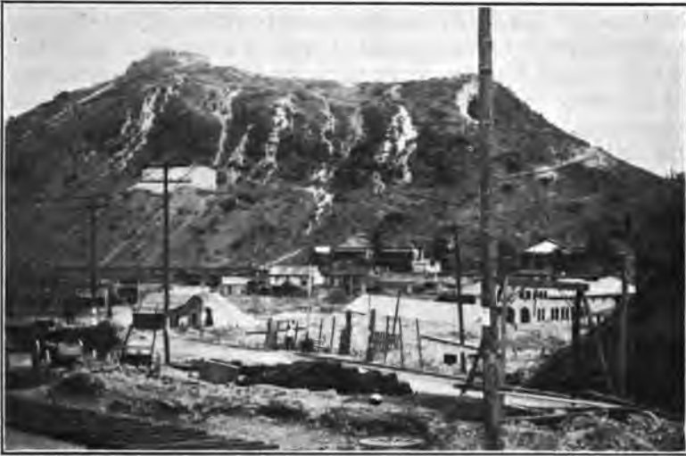
D. ANOTHER VIEW OF SURFACE ABOVE DIVIDEND ORE BODY, CZAR MINE. FILLING ON THE LEFT. COPPER QUEEN C. M. Co.
